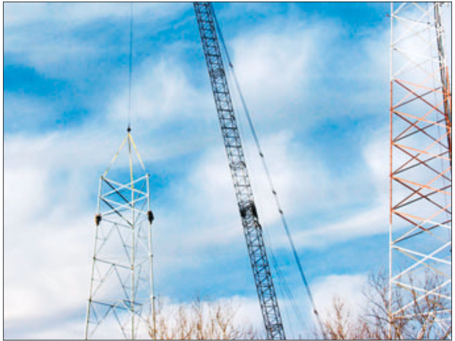
In 2002, work began on the new 800 MHz communications system, which included erecting new towers.
