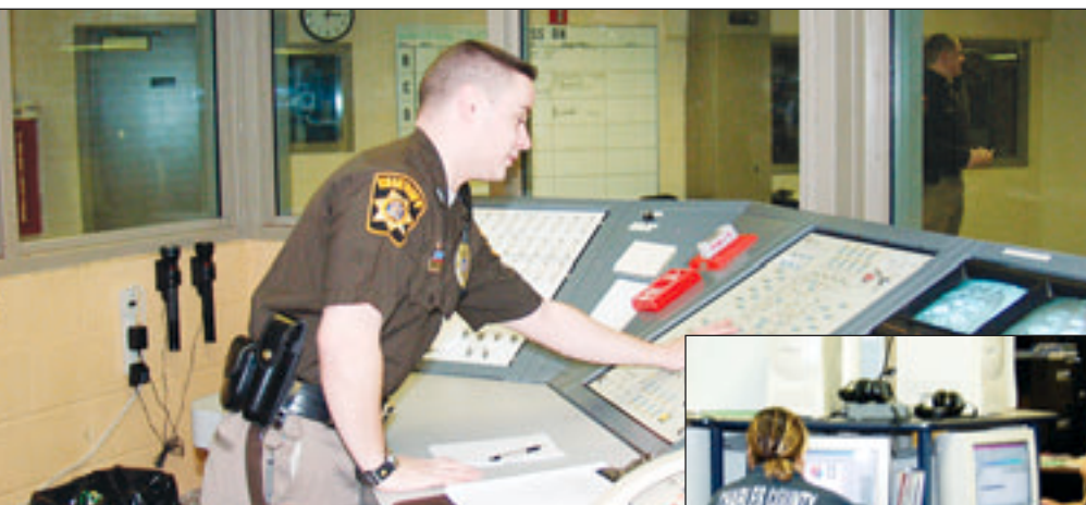
ABOVE: Correctional Officers man the facility's sophisticated control center to maintain safety and security.
